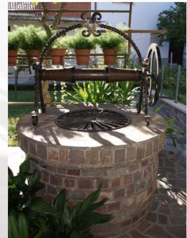
22 constructed by the spouses Filip and Metoda Škvarč in 1985. It is 7 m deep and covered with a cover made of gorged rods.
