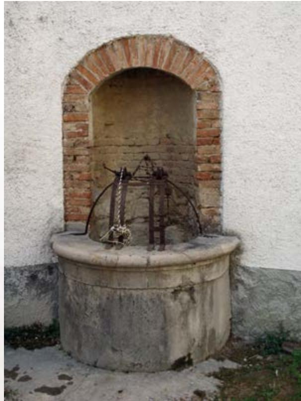
**E**n The owner of the well is Alojz Gorkič, Griči 2, Lower Vrtojba. The 57 house is commonly known as the Lukčevi – Lojze. The well is situated under the outer wall of the house Griči 2 (Gorkič) and by the driveway to the house Griči 4 (Kovic) situated lower downwards. It was constructed before World War I. As the inflow of the water was not strong enough, the well was deepened after the war. It is 22 m deep and covered with a metal cover.
